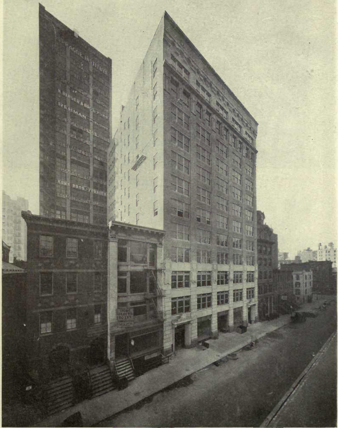
Alan Realty Building, New York, N. Y. Rouse & Goldstone, Architects, Waterproofing & Construction Co., Waterproofing Contractors All under grade foundation work waterproofed with Truscon Waterproofing Paste, Concentrated.
